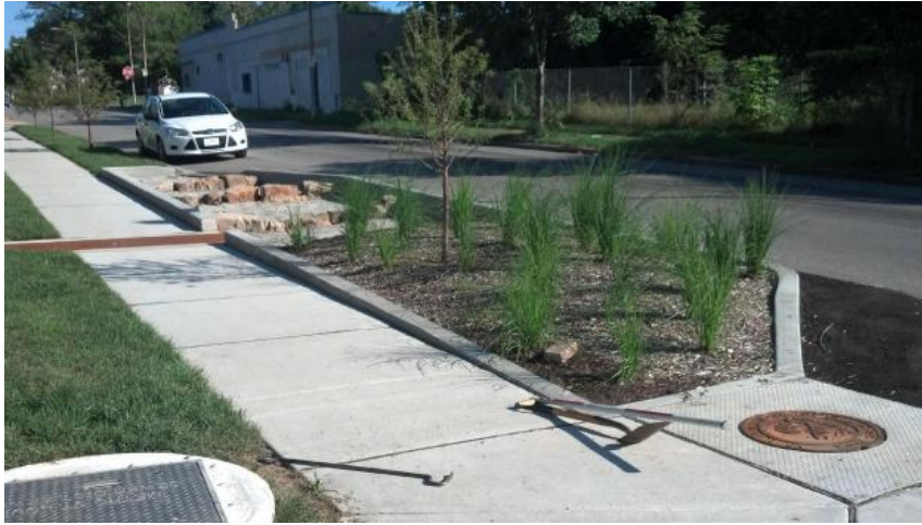
Geraldine Ave. Rain Garden in Mark Twain Neighborhood – Curb bumpout forebay
